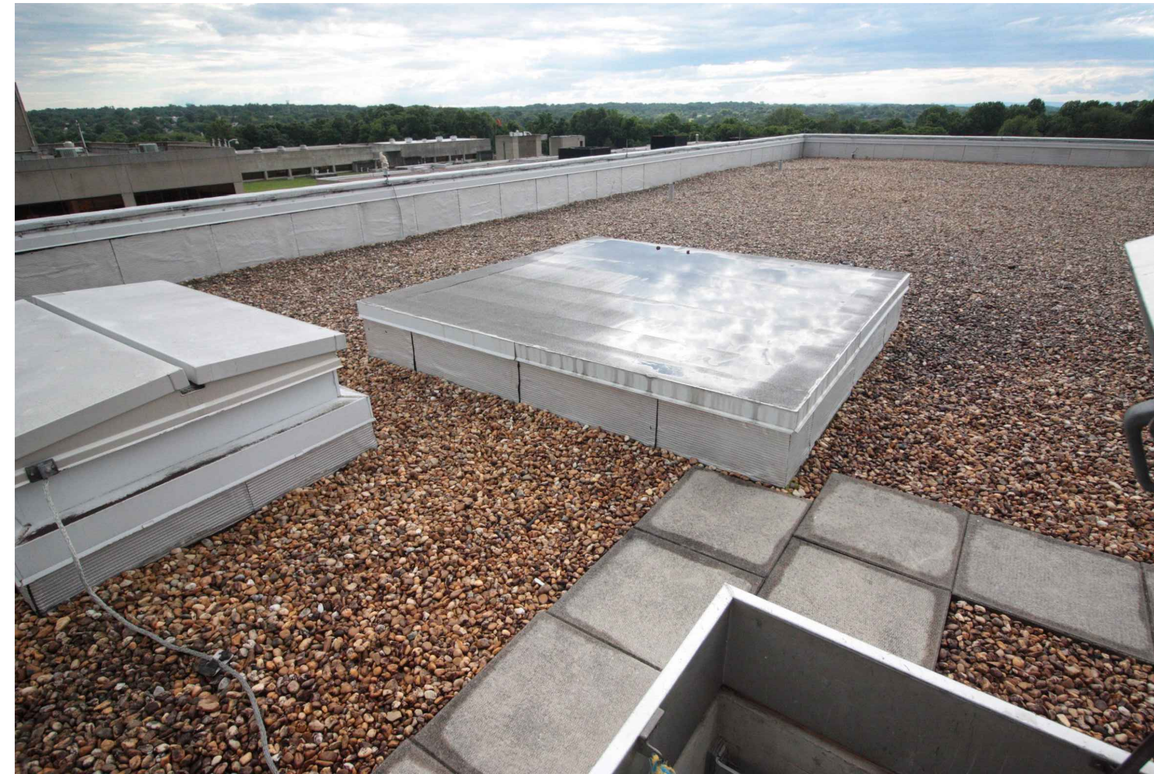
PHOTO 1 - PARTIAL VIEW OF ROOF N.T.S.
