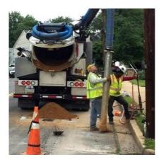
2. Material and Equipment Staging: Prior to the water main installation, the contractor will deliver materials and equipment to the job site and sawcut sections of pavement that will be excavated. Job-site material and equipment storage is required throughout the project. During this time, signs will be placed along the roadway with contact information should there be any questions or concerns.
