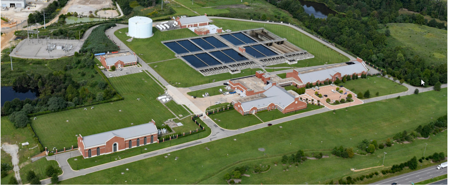
Frederick P. Griffith Jr. Water Treatment Plant, Lorton, Virginia
