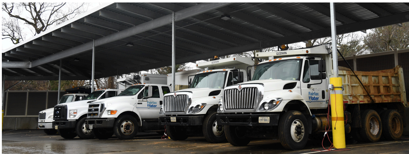
Fleet vehicles will be outfitted with telematics equipment.
