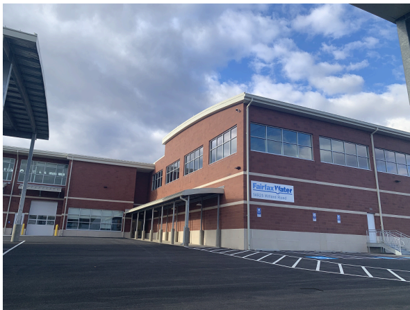
The new Willard Maintenance Facility in Chantilly, VA
