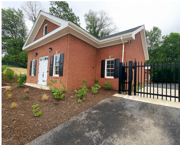
Exterior view of the Sleepy Hollow Pump Station.
