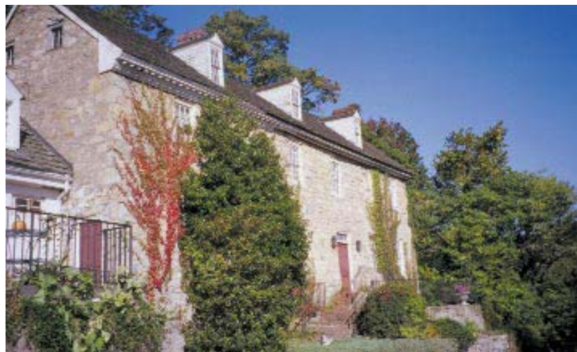
The Rockledge Mansion, inspiration for the pumping station, located in Occoquan, VA.
