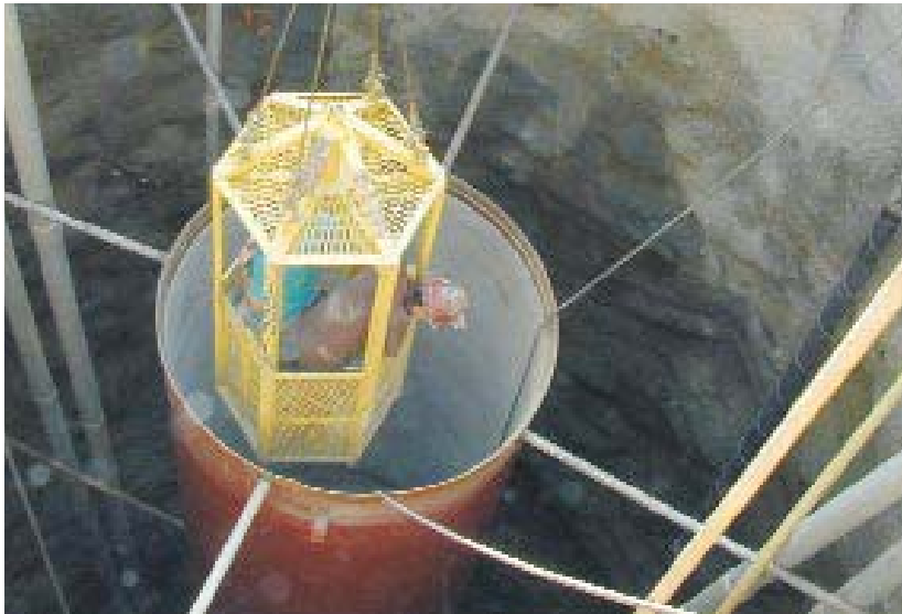
Workers entering 84-inch pipe.
